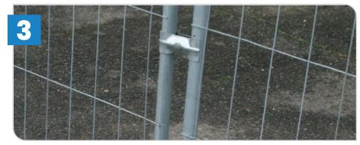
Connect the ends of each barrier together using a coupler.
